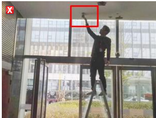
Passenger flow in horizontal direction (wrong)
