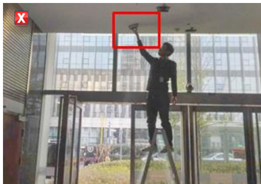
Passenger flow in slant direction (wrong)
