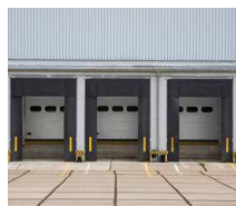
LOADING BAYS & DOCKS
